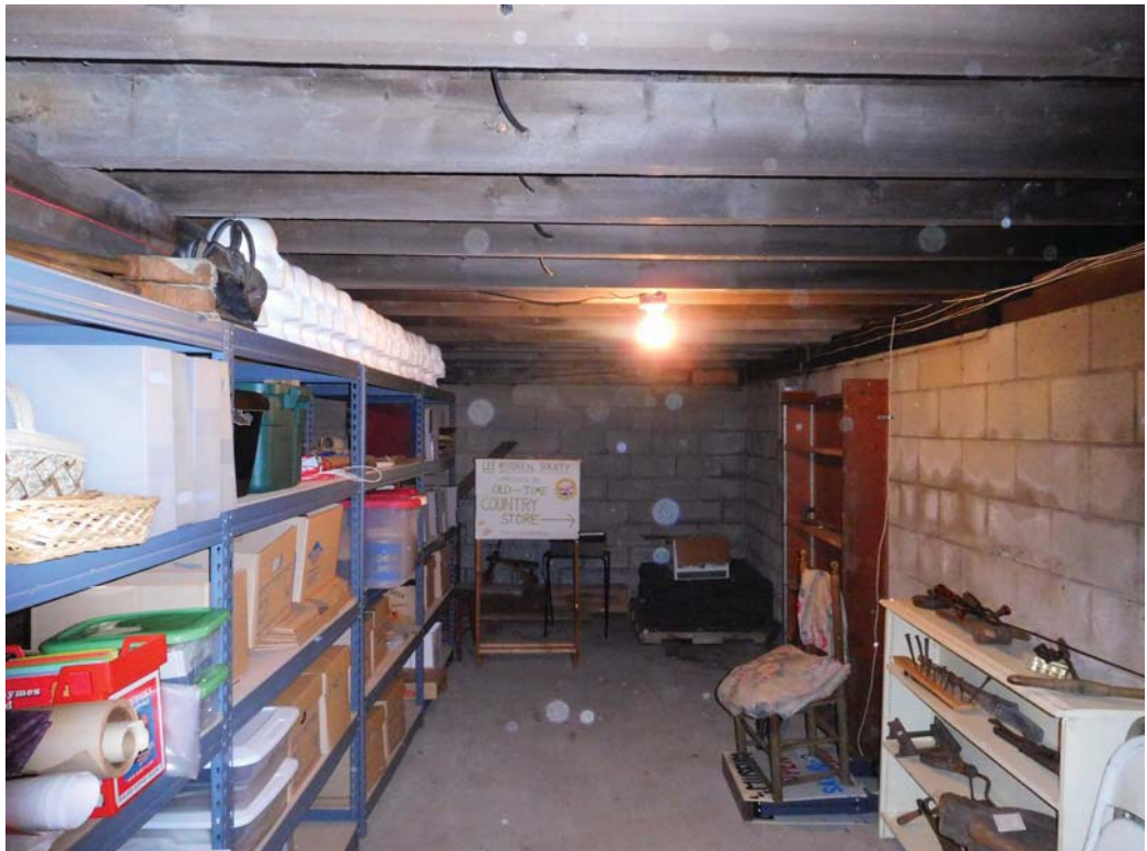
Photo #8 – Shallow joists with sag
