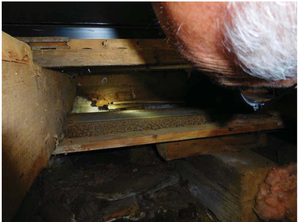
Photo #2 – I-beam support at perimeter
