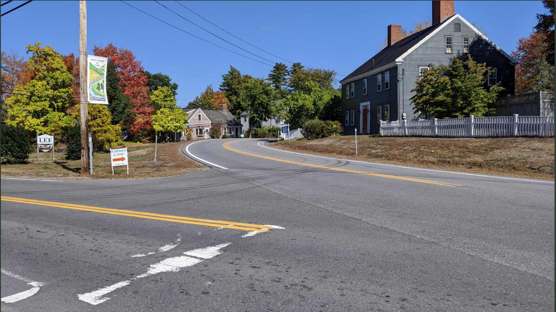
Poor geometry and poor lines of sight (George Bennett Rd. & NH 155)
